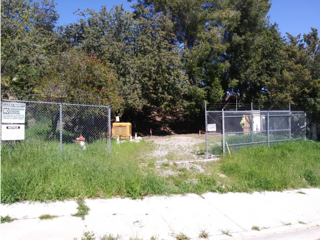
Photo 1. Northeast-facing view from Victory Boulevard of entrance to pump station site.
