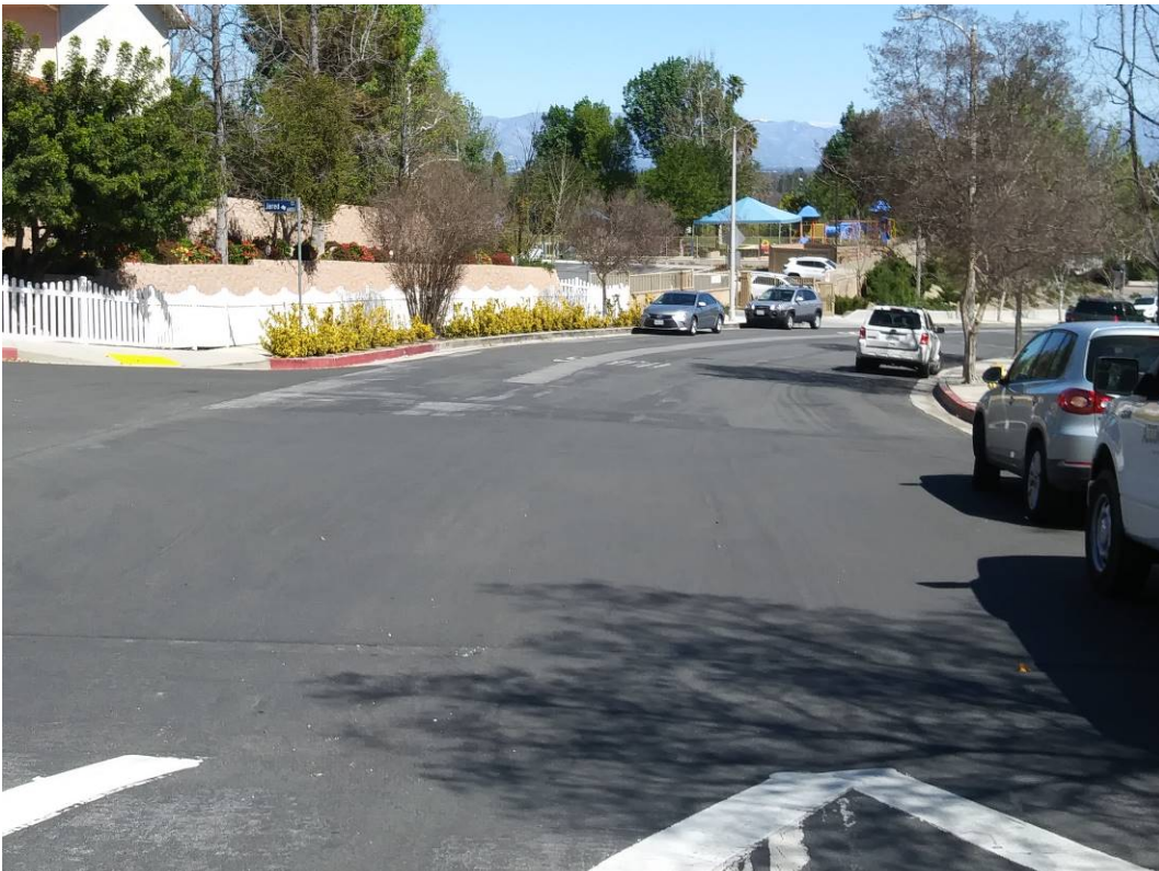
Photo 8. West-facing view along Calvert Street of pipeline alignment. Jared Court enters photo from left.
