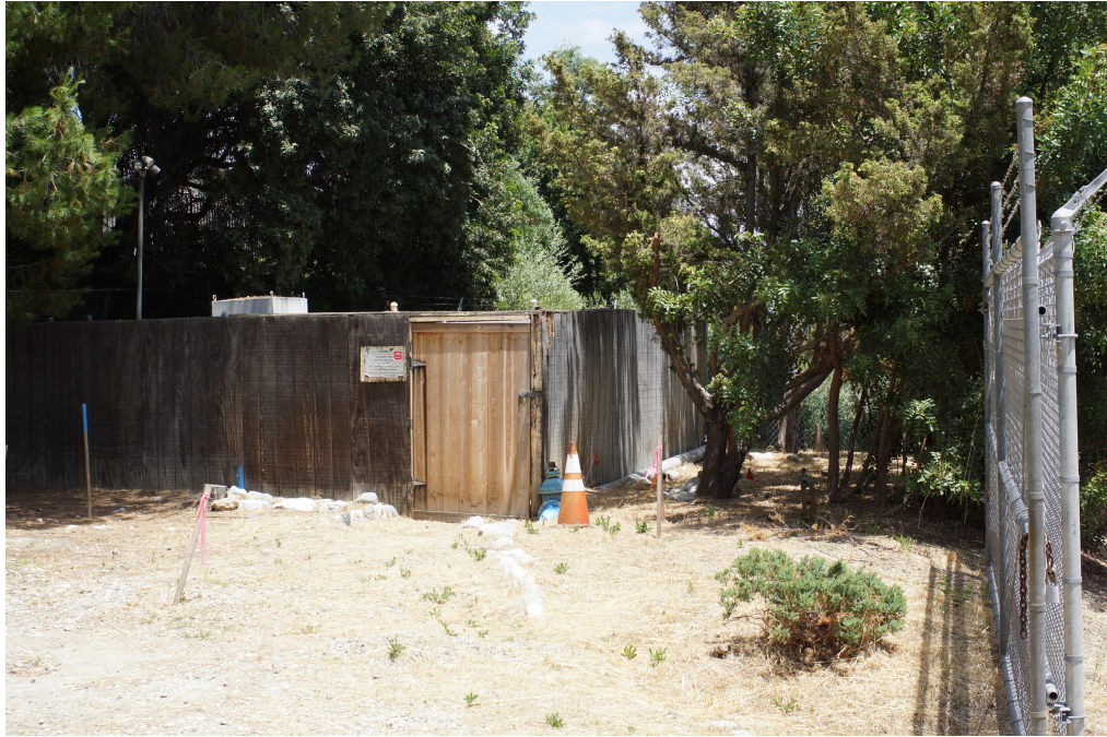
Figure 10: Victory Pump Station, View East.
