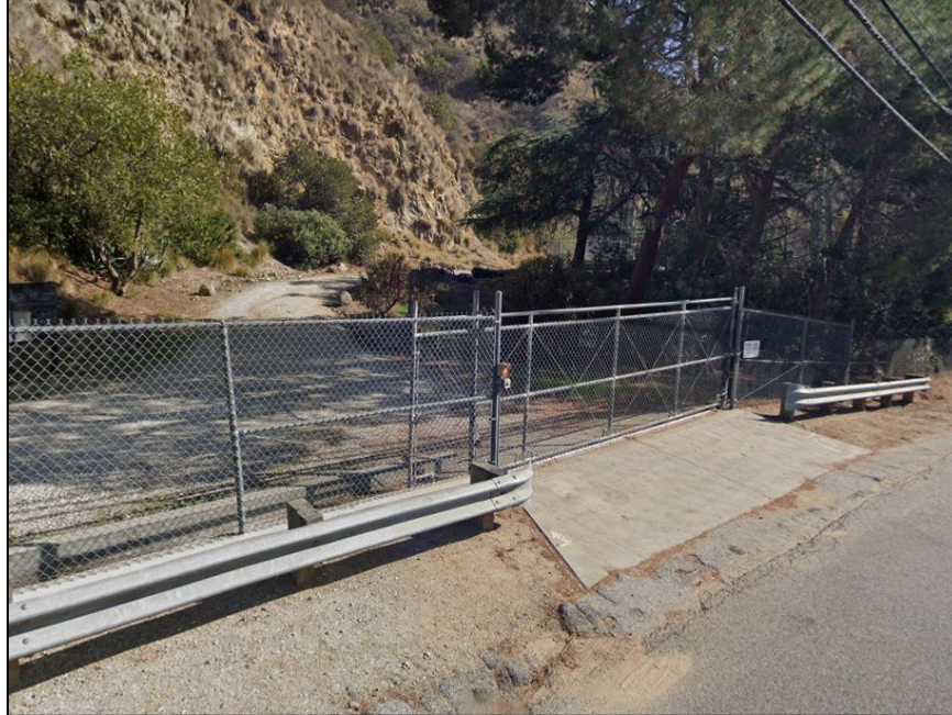
Plate 5: Entrance to the north section of the Nichols Canyon Terminal Tower along Nichols Canyon Road; camera facing southeast. (Google Street View 2021).
