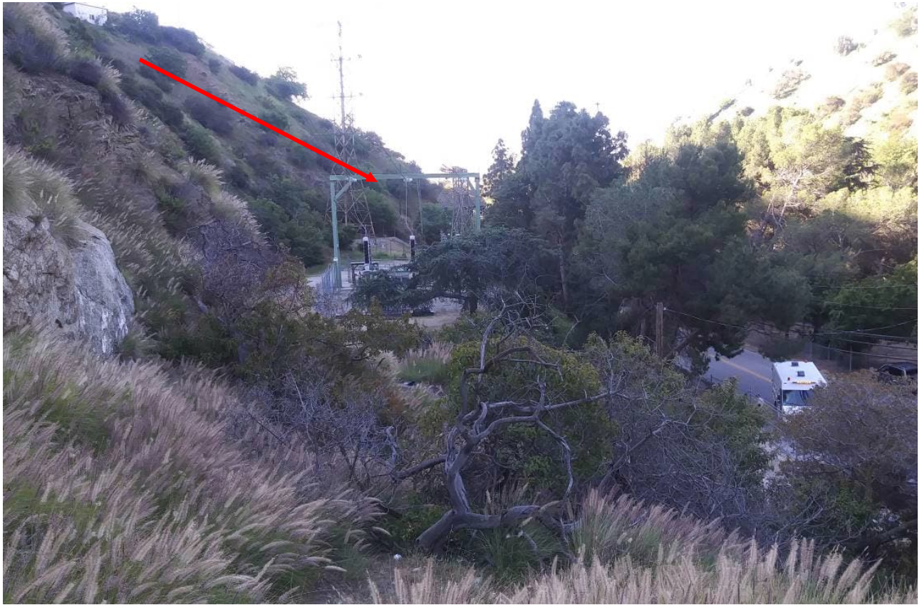
Photo 1: South-facing view of the Nichols Canyon Terminal Tower (red arrow), with Nichols Canyon Road below at left.
