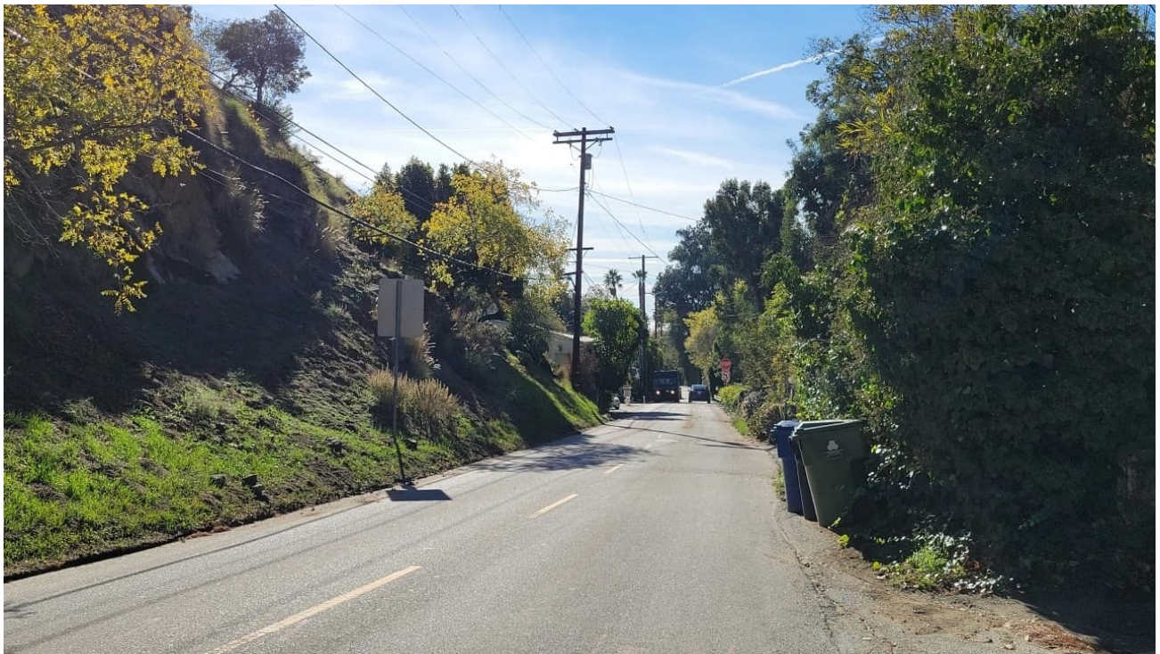
Photo 2: South-facing view along Nichols Canyon Road from the Nichols substation at the northern end of the underground transmission line alignment.
