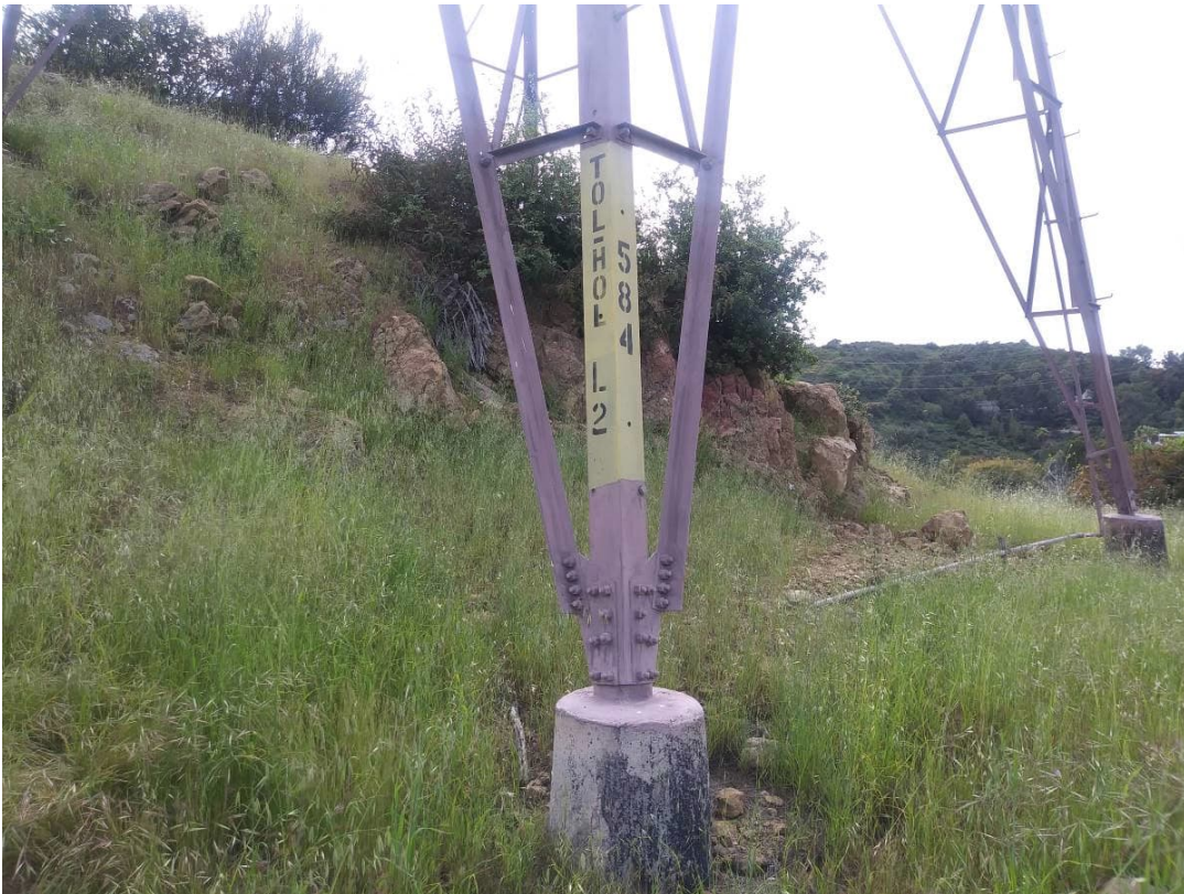
Photo 10: East-facing view of existing Tower 584.
