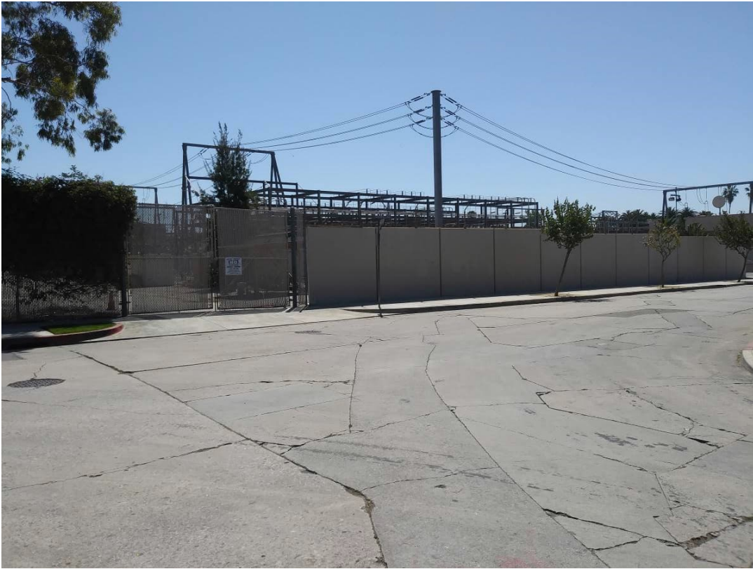
Photo 9: East-facing view entrance to the Hollywood Receiving Station.
