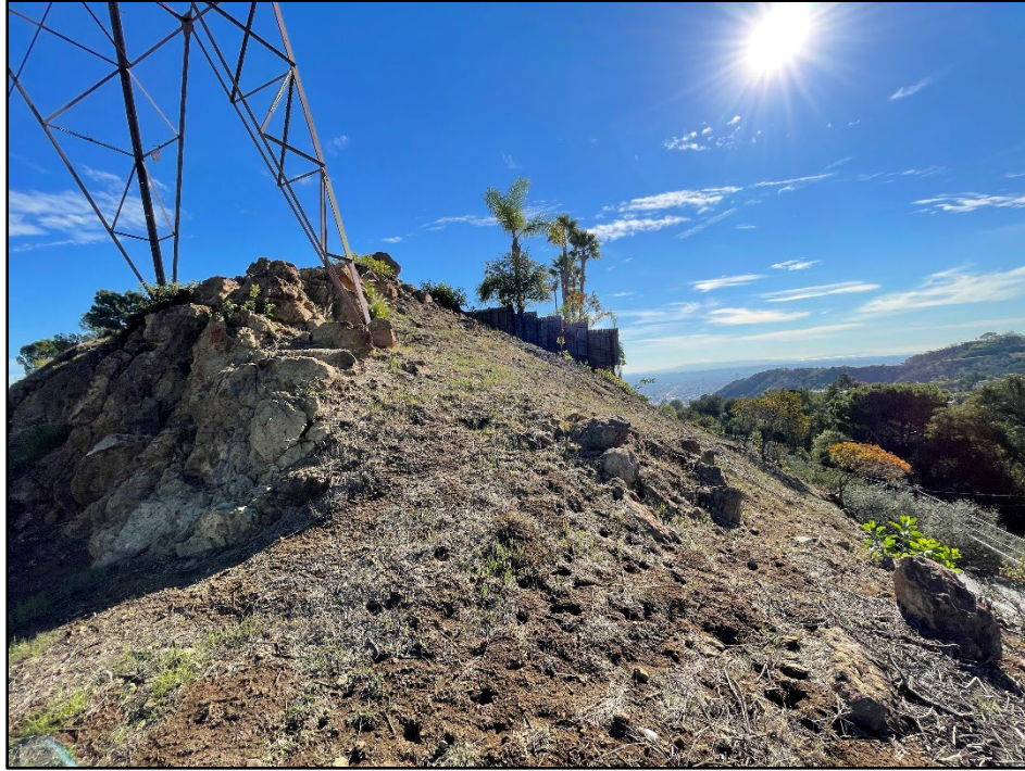
Plate 3: Tower 584 within the Project Work Area.
