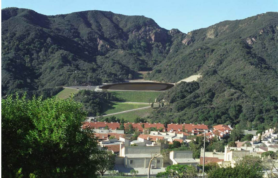
Figure 5: Visual rendering of reservoir with proposed floating cover. Cover would be installed with edges extending up side slopes of reservoir.
