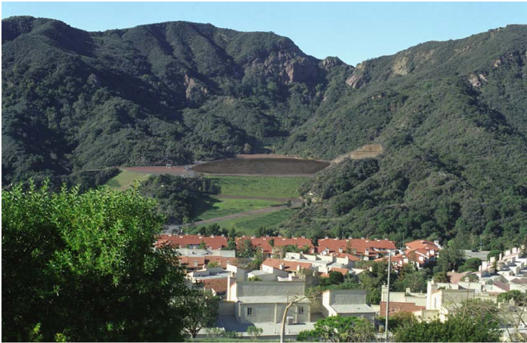
Figure 6: Proposed floating cover with mottling pattern and colored perimeter/approach roads and repaved helipad/parking area.
