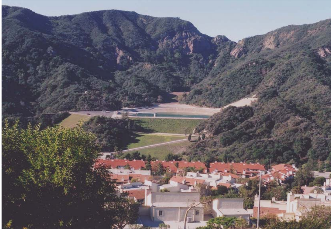
Figure 4: View from 17164 Avenida de la Herradura facing westward (photo date 1/29/03). This perspective shows one of the most prominent views of the reservoir taken from the backyard of a residence within the Pacific Highlands. As such, it is utilized herein as the base image for the evaluation of visual impact and mitigation.
