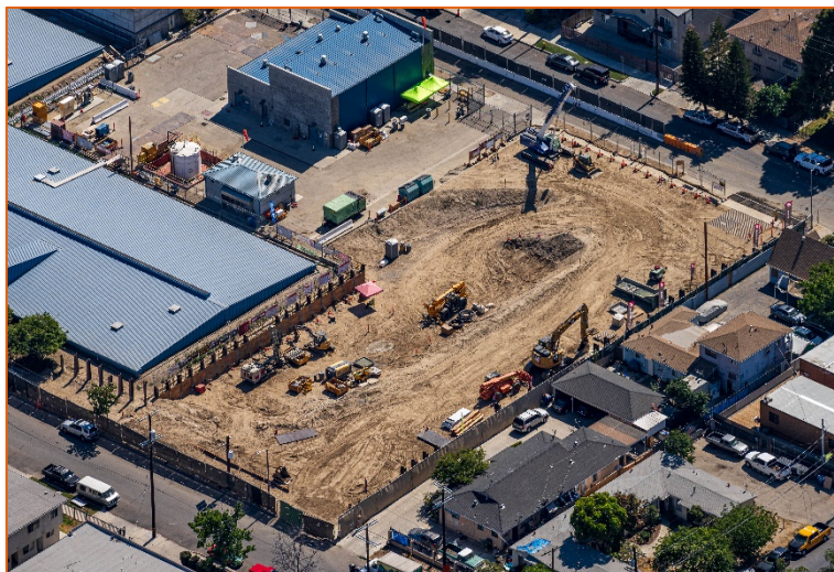
NHC Well Field Facilities Construction
