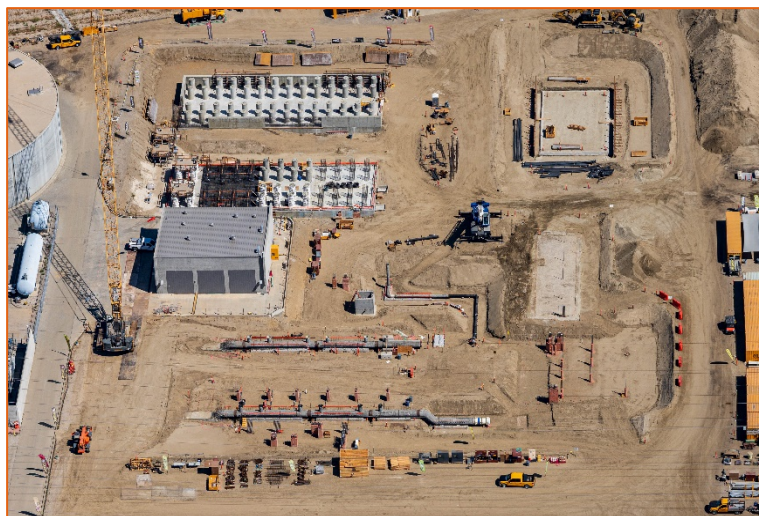
Tujunga Well Field Facilities Construction
