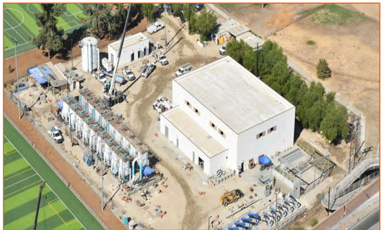
NHW Well Field Facilities Construction
