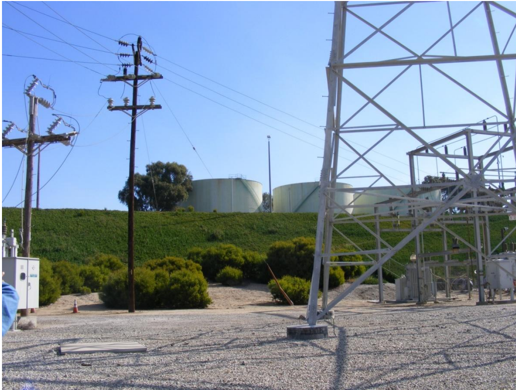
FIGURE 10. FEATURE 3, WATER TANKS
