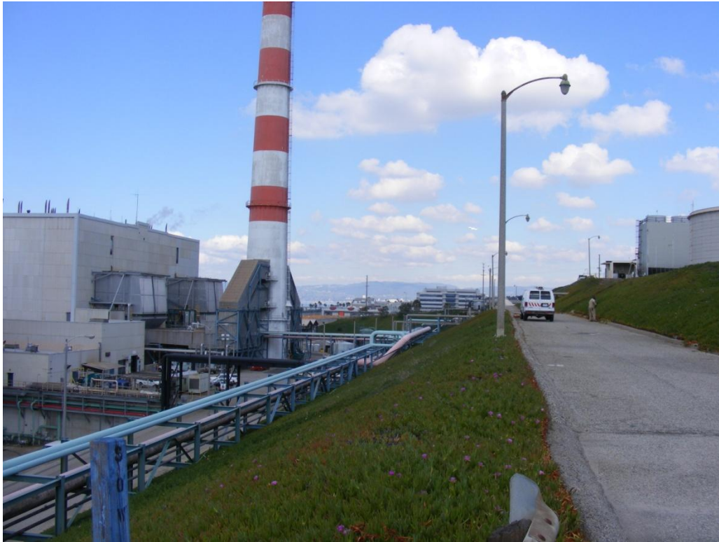
FIGURE 8. OVERVIEW OF FEATURE 1 POWER PLANT AND STACK.
