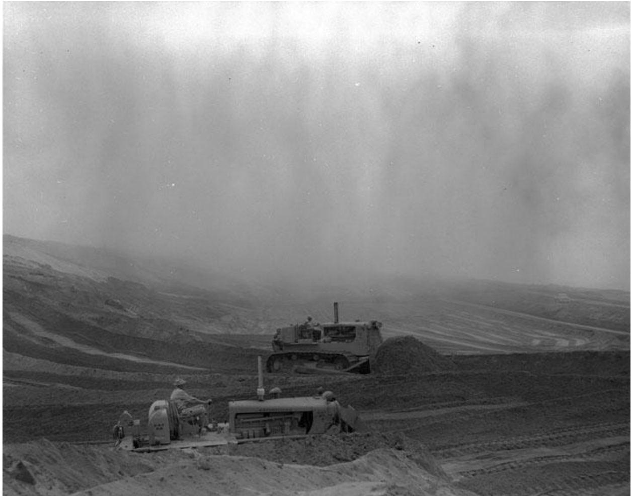
FIGURE 6. BULLDOZERS REMOVING SAND IN PREPARATION OF SCATTERGOOD PLANT CONSTRUCTION, CA. 1958.
