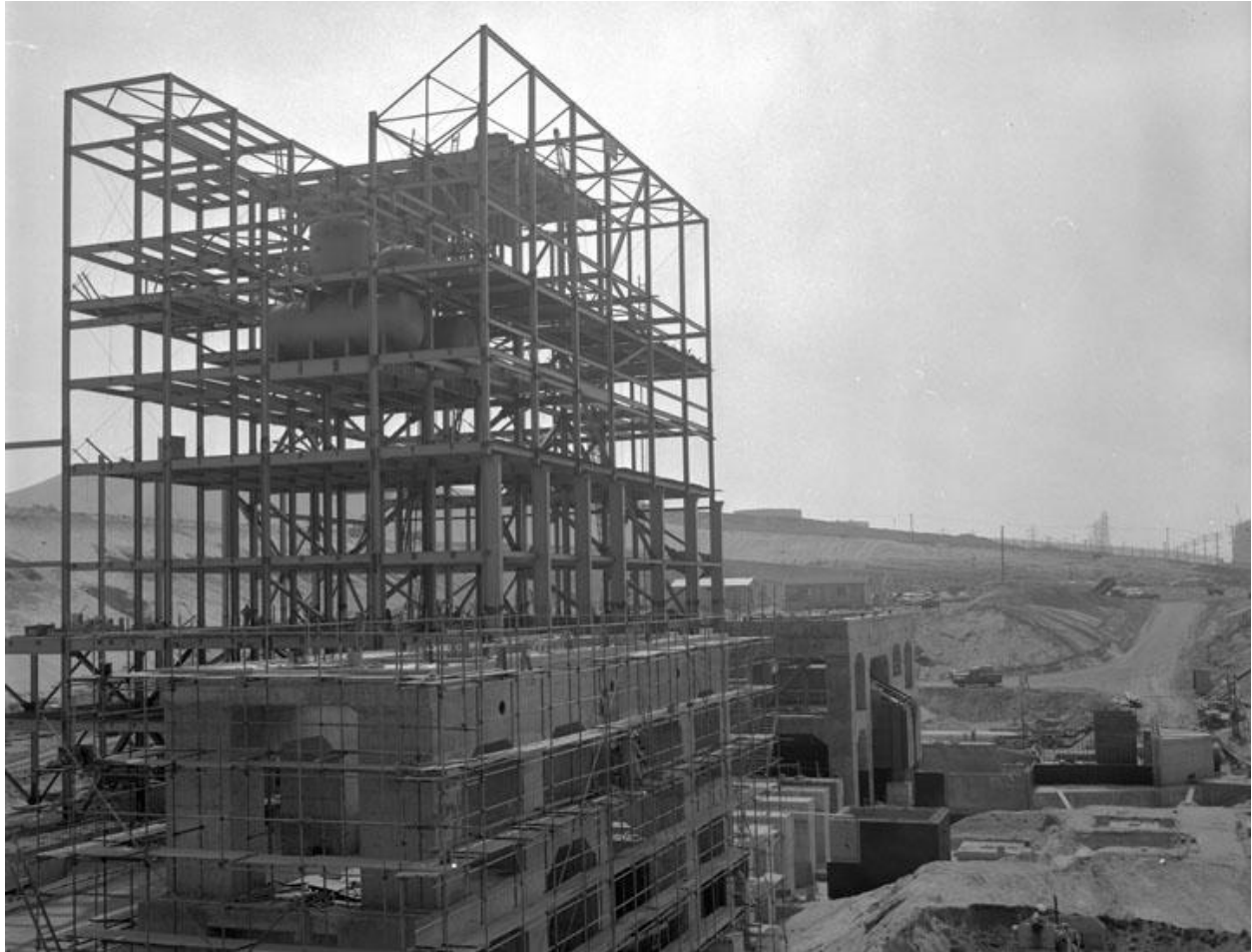
FIGURE 7. SCATTERGOOD CONSTRUCTION IN PROCESS, CA. 1958.
