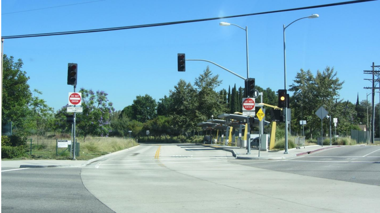
Plate 9. Van Nuys Sherman Oaks Park Segment with Former Southern Pacific Railroad ROW, Current Metroline Busway, View towards Northwest.
