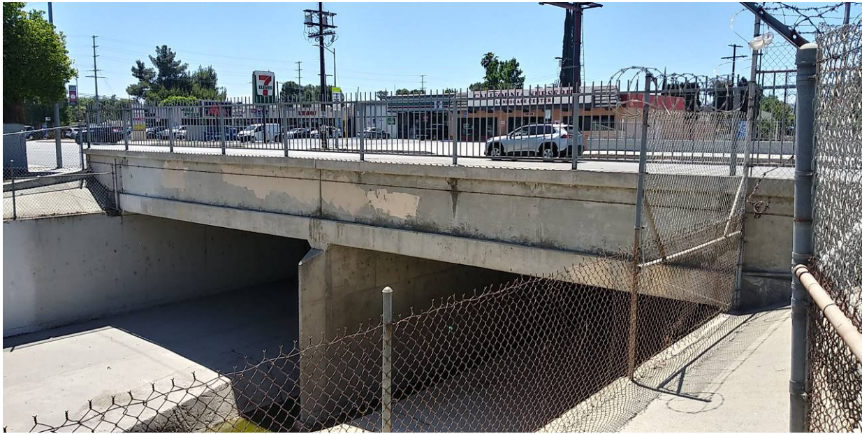
Photo 5: Southeast-facing view of the Aliso Canyon Wash channel under Roscoe Boulevard.
