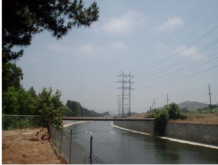
Figure 4-2 Existing Los Angeles River Pipe Bridge
