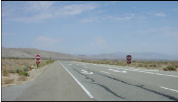
Photograph 5 - Looking north along the west side of State Route 14 from Pine Tree Canyon Road
