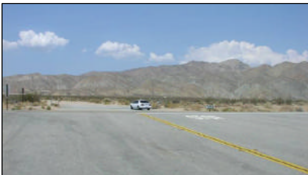
Photograph 7 - Looking west from the State Route 14 median at Pine Tree Canyon Road
