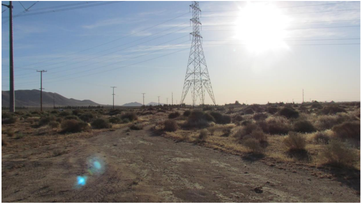
Photograph 1: Representative view of the LADWP easement facing east from the easement toward the Site. The Site is located beyond the transmission tower in photograph.
