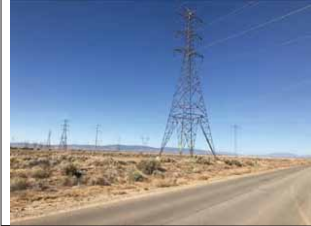
View of the Property, camera facing southwest from Rosamond Boulevard.
