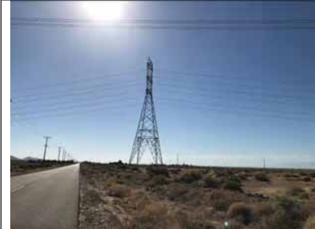
View of the northern portion of the Property along Rosamond Boulevard, camera facing east.
