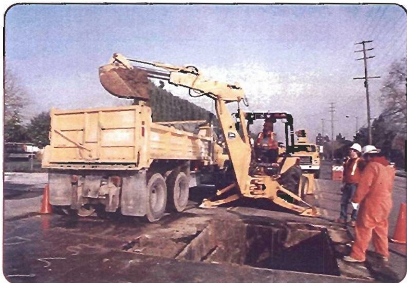
Water system dump truck and backhoe.
