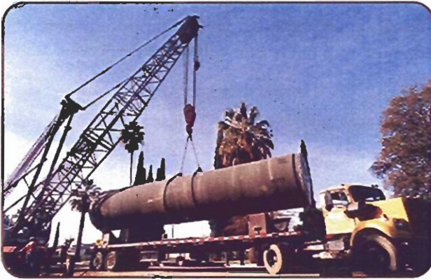
Trunk line being installed on Sepulveda Boulevard
