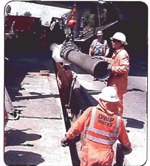
Water system crews installing mainline.
