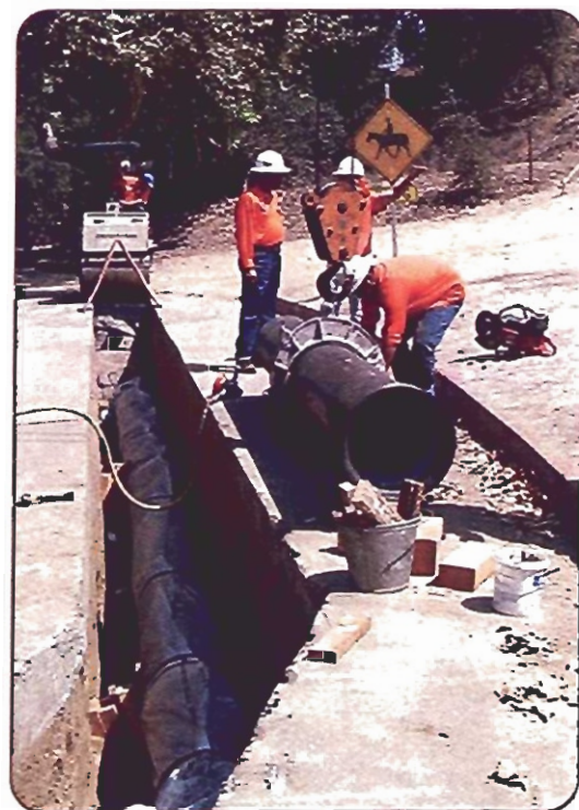
Crews installing main lines in Griffith Park
