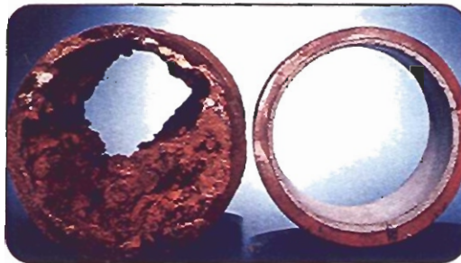
Pipe before and after cement lining treatment.
