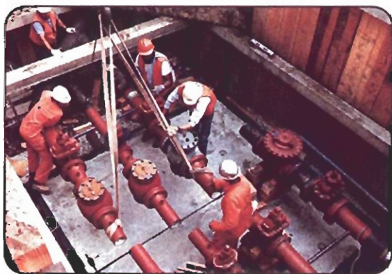
Crews installing a regulator station.
