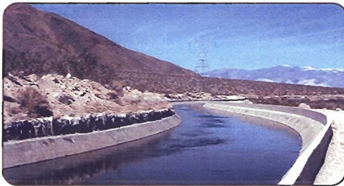
Los Angeles Aqueduct
