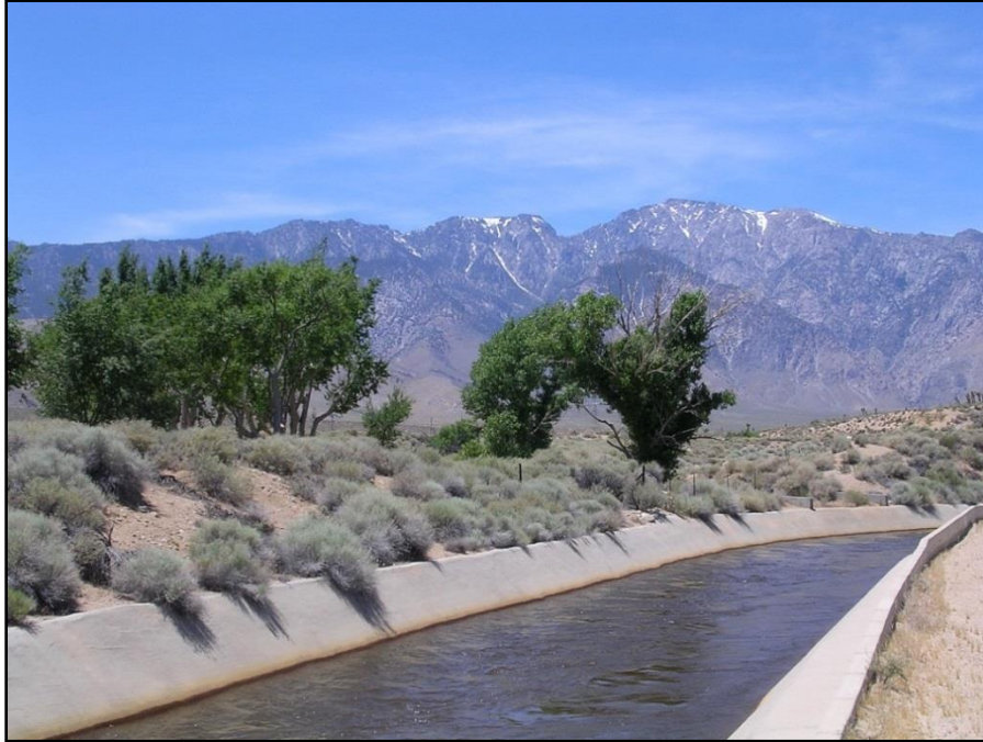
Figure 4-14. LAA1 as a concrete-lined, open canal on western side of the Project Site.
