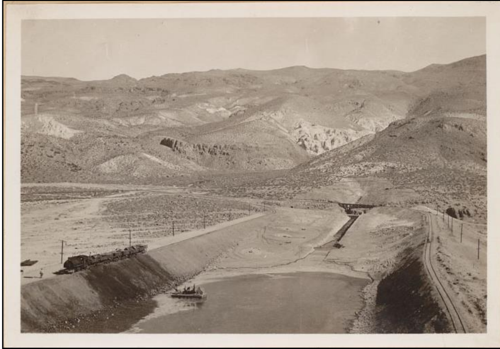
Figure 2-8. Construction of SHD, 1911.
