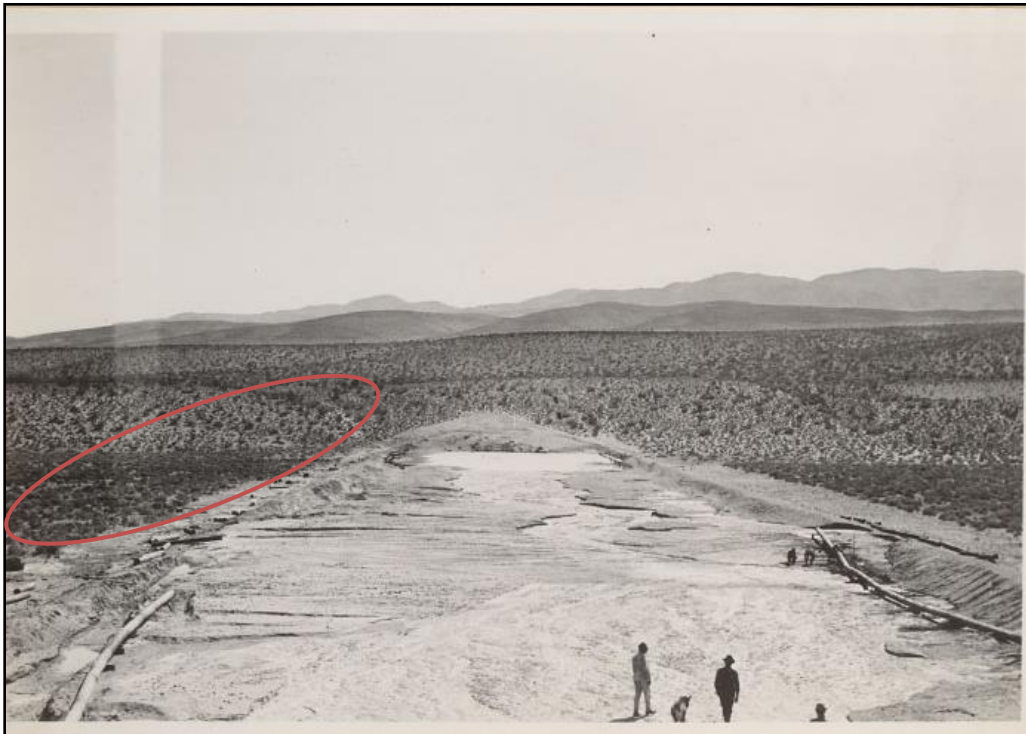
Figure 2-9. Construction of NHD, facing east.
