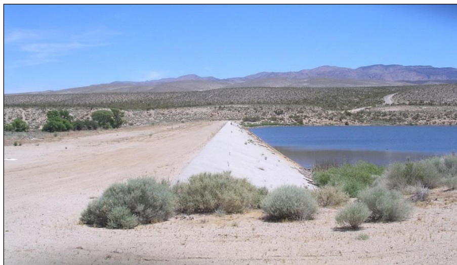
Figure 4-15. NHD overview, facing east.
