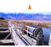
The LADWP will modify the Los Angeles Agueduct structure and replace the existing radial gate with a new, automated gate that allows reliable control of river water from the aqueduct to the Lower Owens Riverbed.
