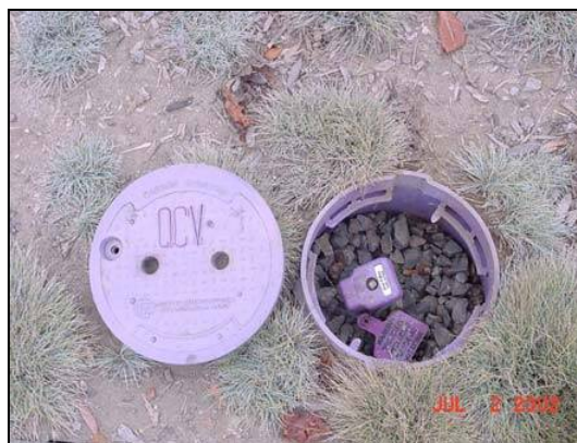
Tagged quick coupler and valve box
