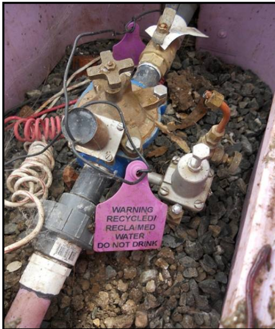
Tagged remote control valve
