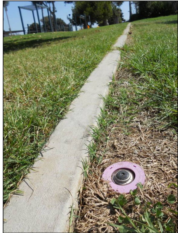
Concrete "mow strip" separates potable water and recycled water irrigated areas
