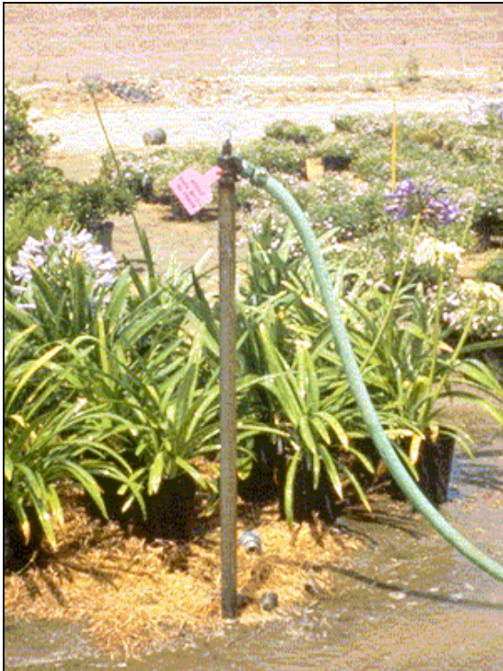
Hose bibs may only be used with recycled water in areas where they cannot be accessed by the general public (such as this commercial nursery), and even those must be properly labeled.
