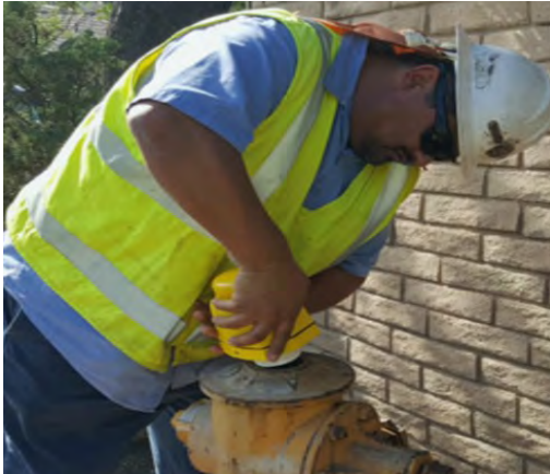
Installation of a Pressure Logger
