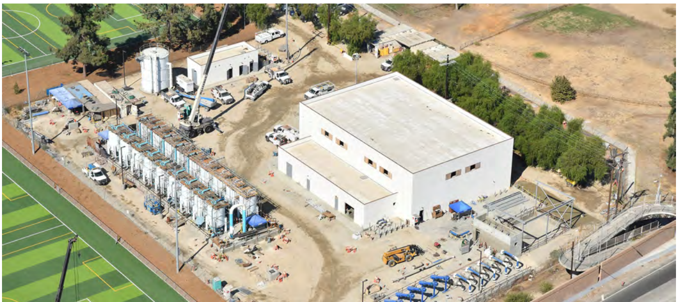
North Hollywood West Groundwater Remediation Project
