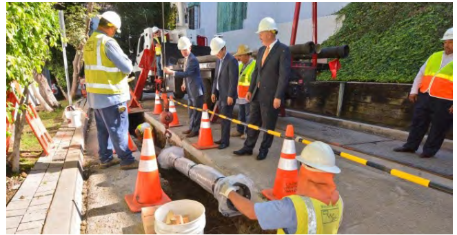
Mainline Replacement on Valley Oak Drive
