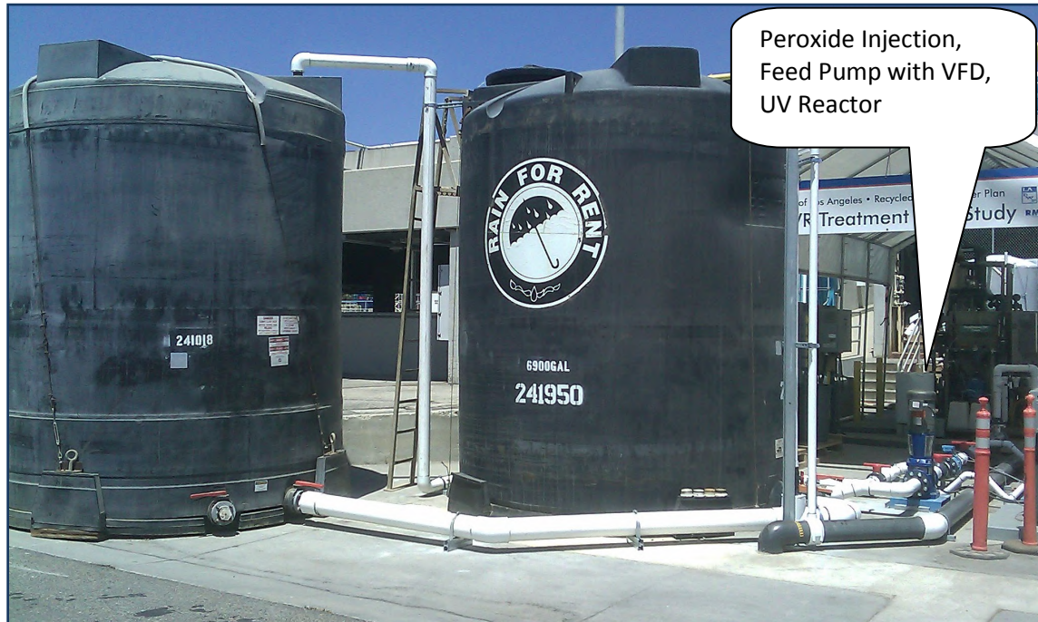
Figure 2-8: UV/Peroxide Equipment for Phase 2 Testing
