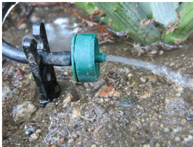
DRIP TUBING WITH 1 OR 2 DRIP EMITTER(S) PER SHRUB
