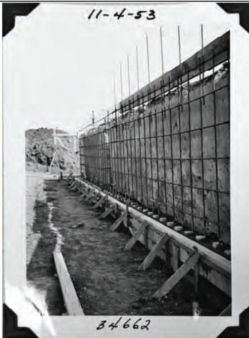
West Los Angeles Headquarters, Building 2 (warehouse), north end of fill showing footing and reinforced steel for foundation wall ; November 4, 1953 (LADWP No. 34662)
