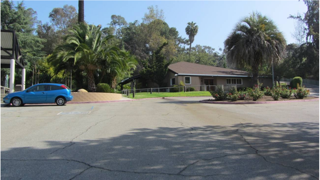
Figure 3.1-2: Existing view towards northwest of Grace E. Simons Lodge within Elysian Park
