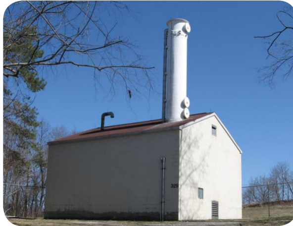
Air stripper and treatment building
