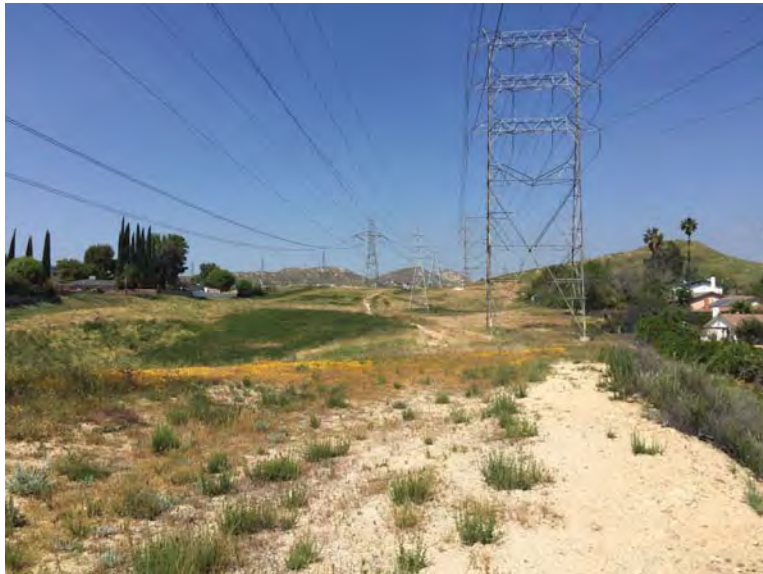
Northern portion of the alignment, where the alignment crosses a single-family residential neighborhood in the City of Santa Clarita, north of Bouquet Canyon Road.
