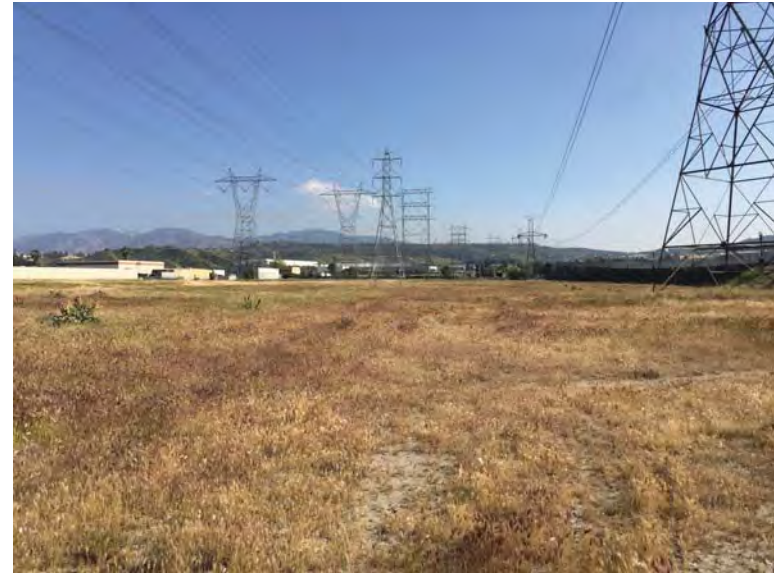
Center portion of the alignment, where the alignment crosses an industrial area in the City of Santa Clarita, just south of the Santa Clara River.
