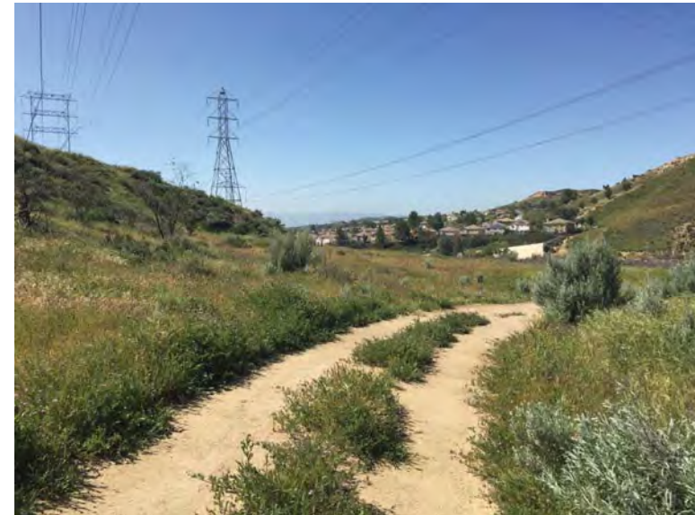
Northern portion of the alignment, where the alignment extends from open space to a single-family residential neighborhood in unincorporated Los Angeles County, north of the City of Santa Clarita.
