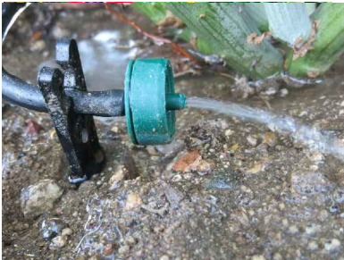
DRIP TUBING WITH 1 OR 2 DRIP EMITTER(S) PER SHRUB
