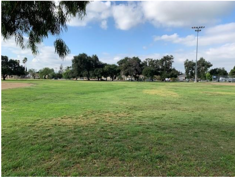
Photo 7. Facing south at baseball fields where underground infiltration gallery will be installed.
