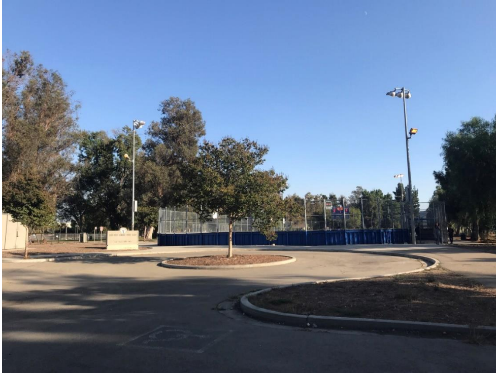
Photo 31. Facing south at skating rink with coast live oak tree in the parking lot where underground infiltration gallery #2 is proposed for installation.
