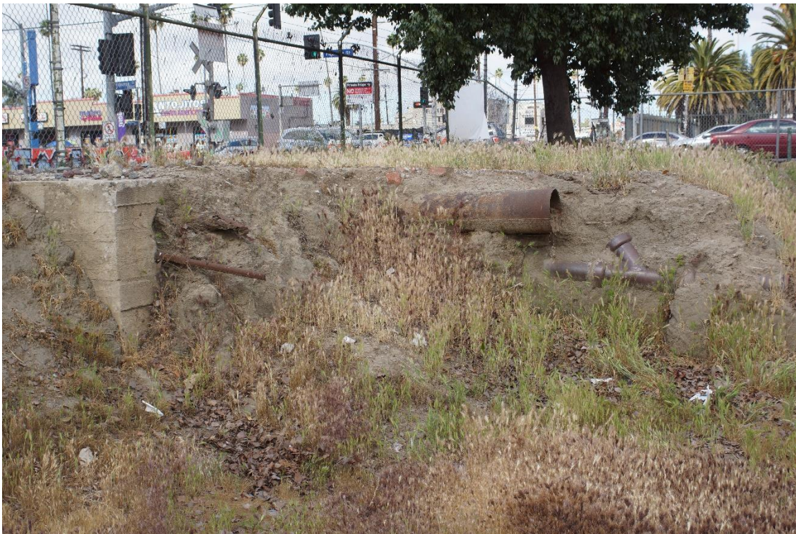
Plate 3: Building Foundation, View Southwest.
