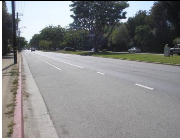
View towards west on San Vicente Boulevard, near Bristol Avenue
