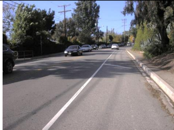
View towards east on Entrada Drive, near Stassi Lane
