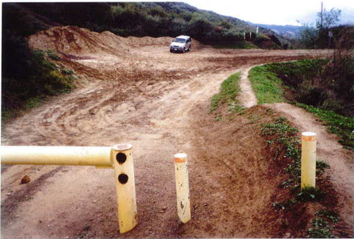
Photo 4: View facing south of Project Site (half-way point and end of public vehicle access).
