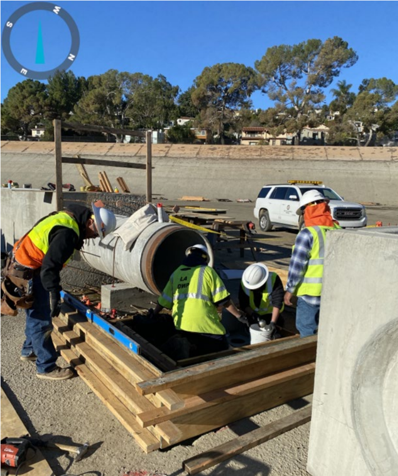
Left Photo: 36" pipe concrete encasement inside Ivanhoe
