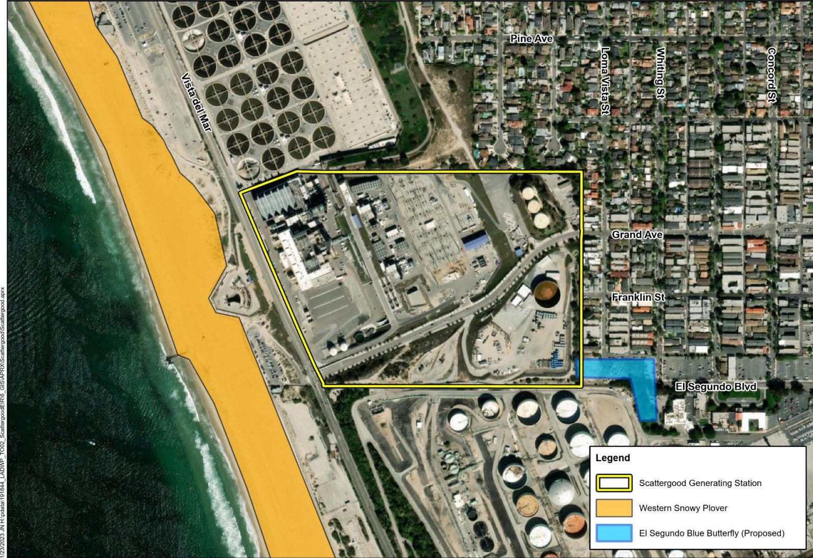
SCATTERGOOD GENERATING STATION UNITS 1 AND 2 GREEN HYDROGEN-READY MODERNIZATION PROJECT
