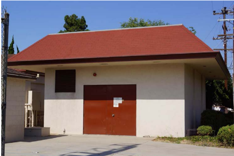
Plate 13: 99th Street Wells Pumping Station Building 2, View Facing Southwest.
