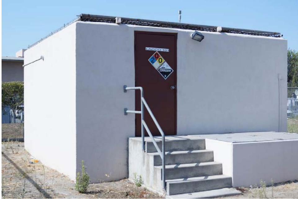
Plate 16: Building 5, Oblique View to Southwest.
