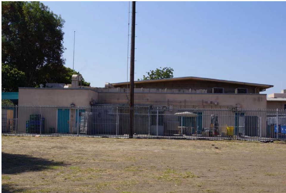
Plate 22: 99th Street Elementary School Building 3, View Facing South
