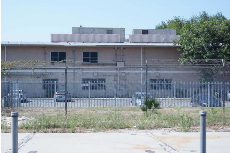
Plate 21: 99th Street Elementary School Building 2, View Facing South
