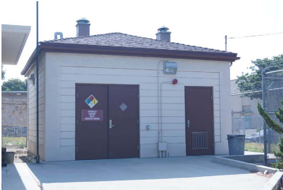
Plate 17: Building 6, North Façade, View to Southwest.
