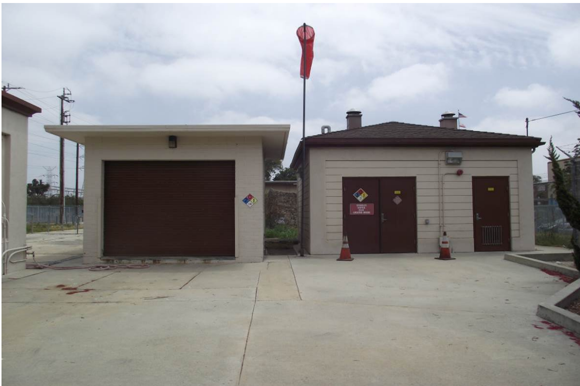
Photo 4: East-facing view of existing chloramination building at left and fluoridation building at right.
