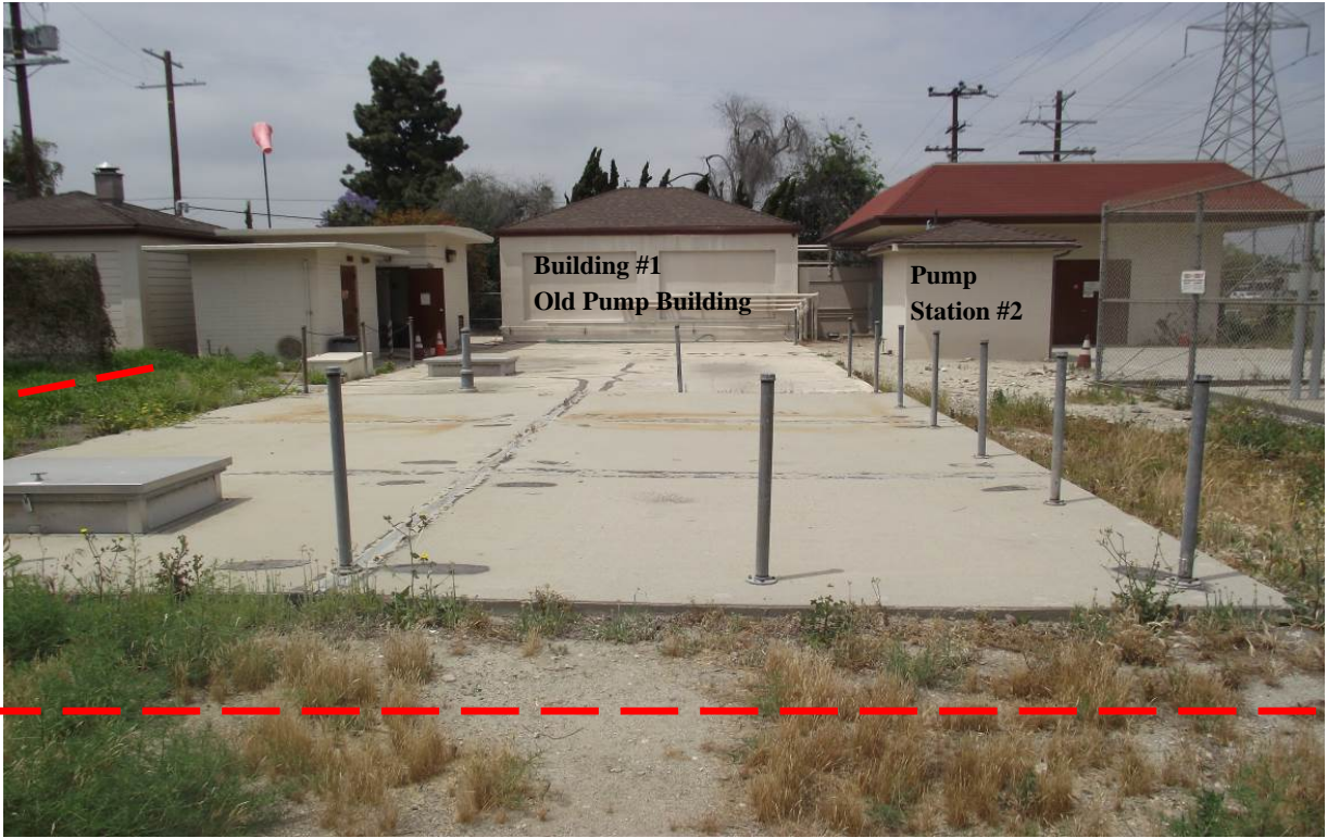
Photo 5: West-facing view of existing structures with proposed pipeline alignment (red-dashed line).
