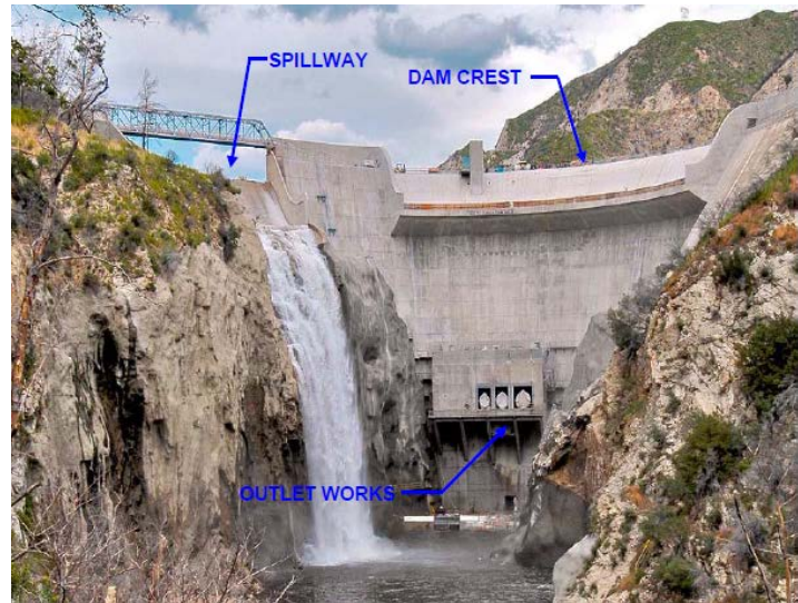
Big Tujunga Dam and Reservoir
