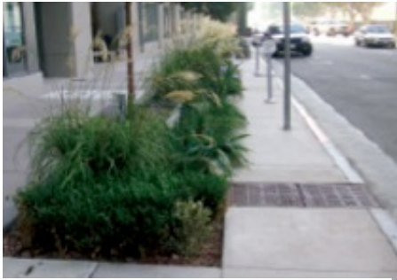
Hope Street Stormwater BMP
