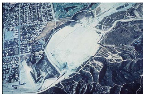
Lopez Dam and Basin
