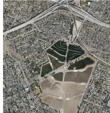
Pacoima Spreading Grounds
