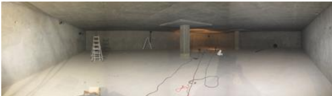
Figure: Inside the Cistern at the Santa Monica Public Library
