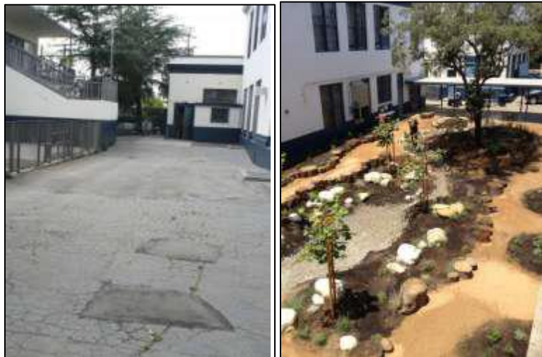
Figure: LAUSD has implemented asphalt removal; Before/After on at Main Street Elementary School.
