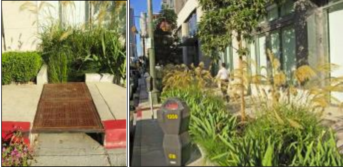
Figure: Example Stormwater Planter on Hope Street in Downtown Los Angeles, CA (photo courtesy of California Regional Water Control Boards, 2014)
