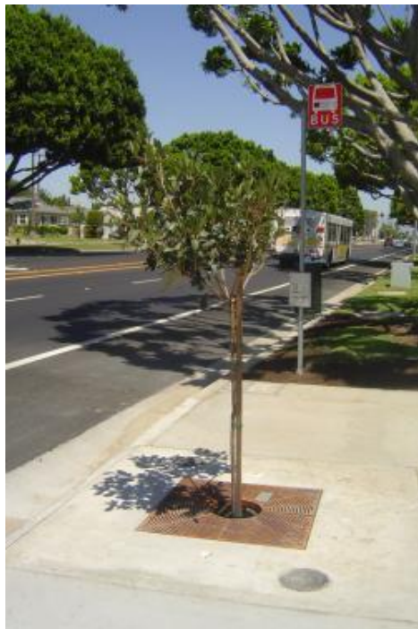
Figure: Example Tree Well installed in Lakewood, CA and Tree Well Schematic Design showing Filterra® Internal By-Pass - Curb (photos courtesy of Filterra, 2014)
