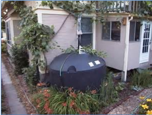
Figure: Cistern on Single-Family Homes
