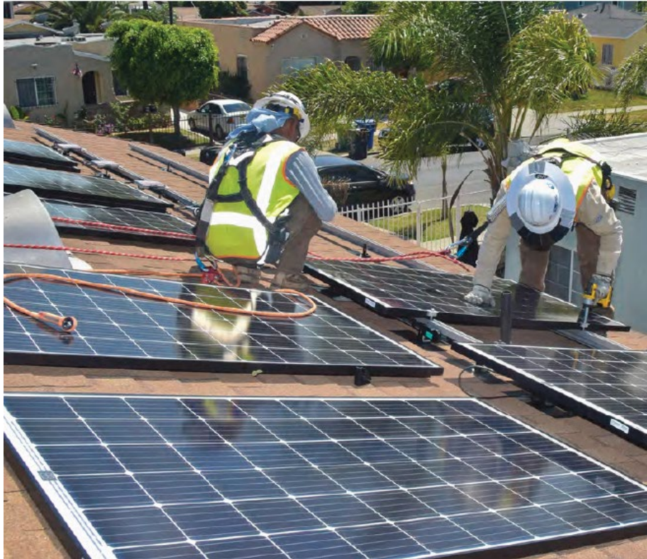
Figure 2. Installation of local rooftop solar.
