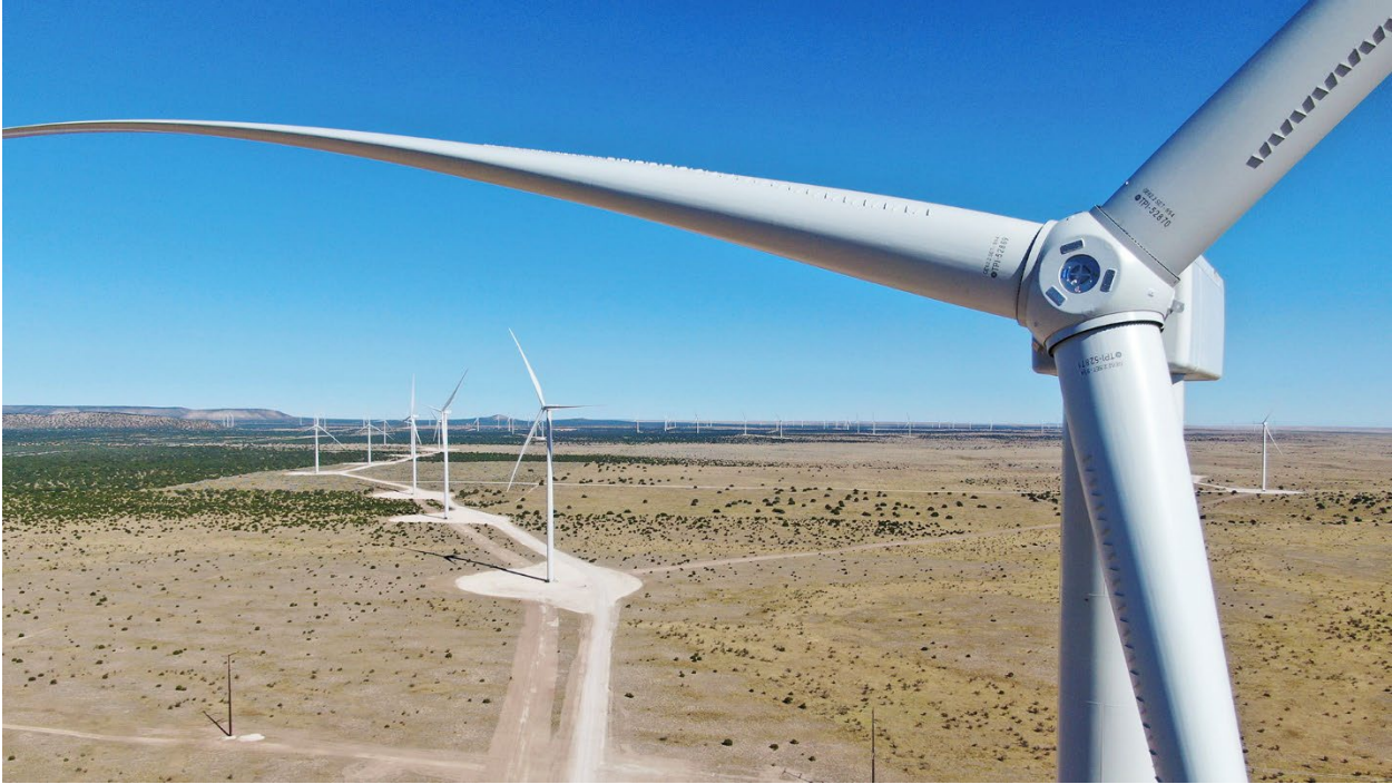
Figure 4. Red Cloud Wind Project, located in New Mexico.
