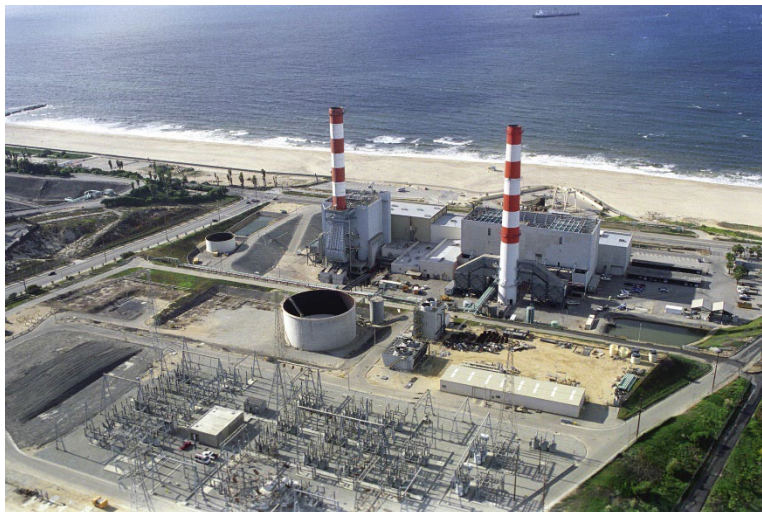
Figure 1-5. Scattergood Coastal Generating Station.
