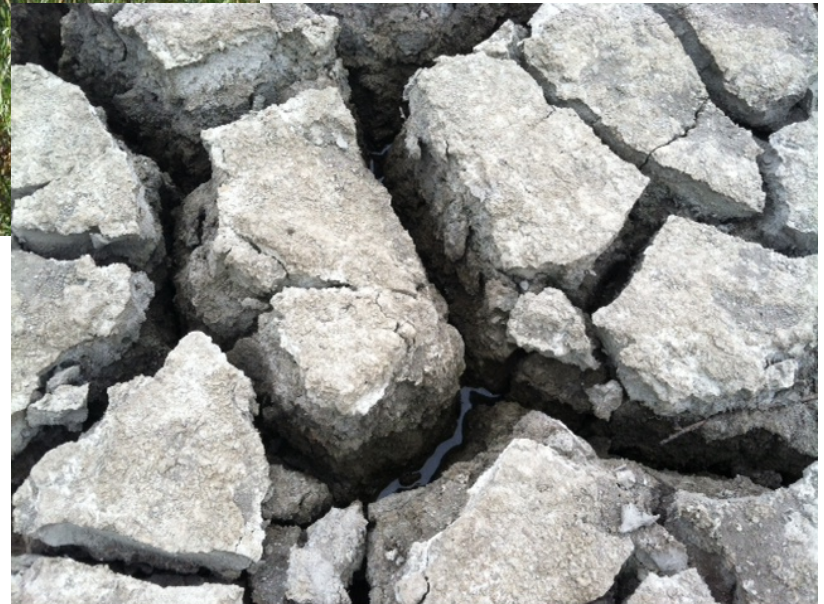
Water below the silt
