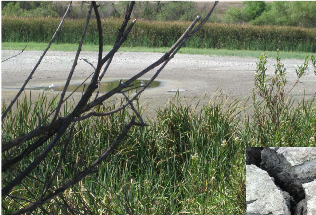
7-29-15: Level of Silt
